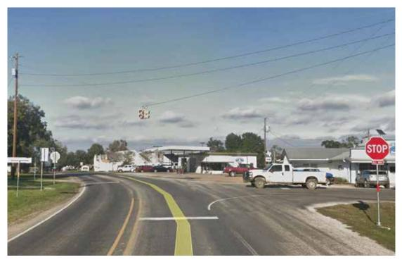
Description: The intersection of 237 and Main Street utilizes a flashing stop signal. Cars from both roads stop at the intersection. Speeds are reduced before entering Round Top, allowing drivers to become more aware of pedestrians and slower-moving traffic in town.
